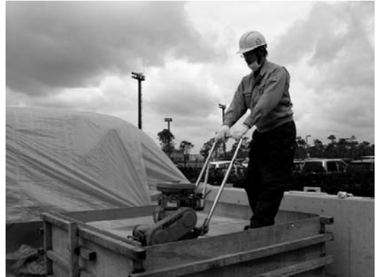
写真2.7 地盤の密度検定 Photo 2.7 Examination of compaction.
