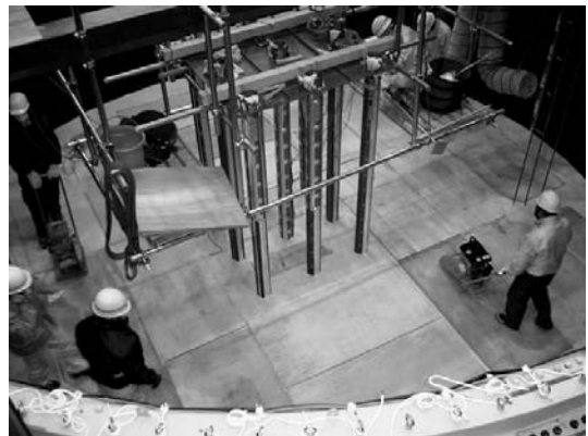
写真2.8 地盤の作製 Photo 2.8 Compaction of sand.
