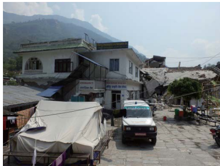
写真 19 病院の被災状況(全景) Photo 19 Damage of the hospital in Khadichaur.
