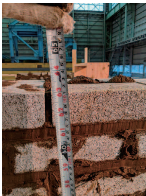
写真11 目地の状況 Photo 11 Condition of joint material.
