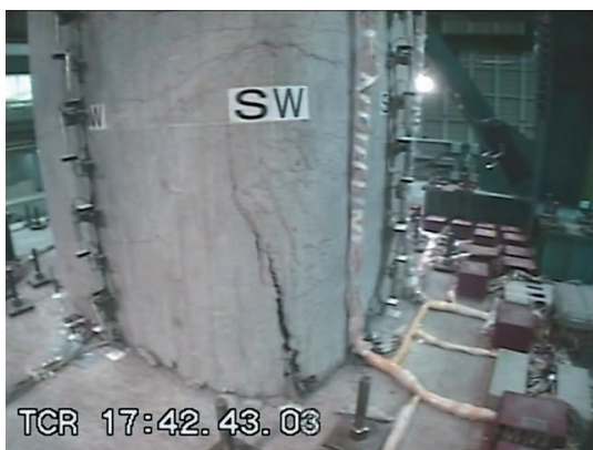
(a) SW corner
