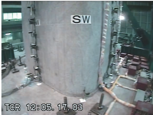
(a) SW corner
