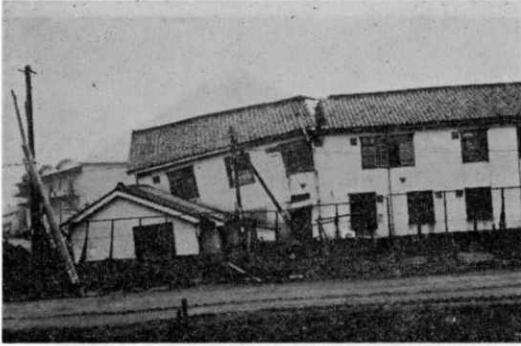
写真-11 建物接続部の被害(海上保安本部・中央埠頭) Damage to the joints between the structures of the same story.
