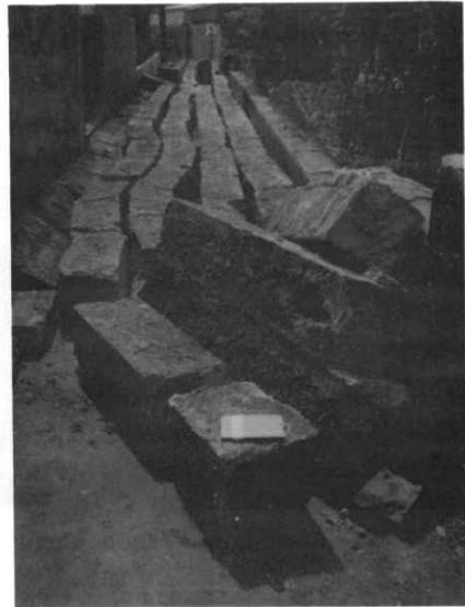
Fig. 13-1. Falling-down of a stone wall at Kyomachi.
