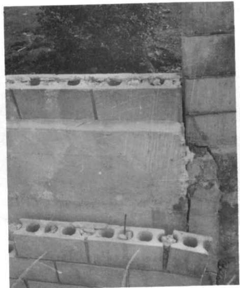
Fig. 13-2. Damage to a concrete-block wall incompletely constructed at Kyomachi.
