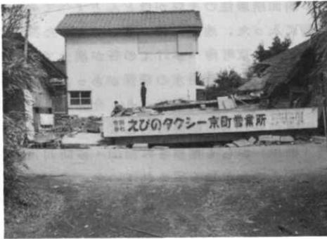
Fig. 10. The completely destroyed concrete-block house of the Kyomachi Taxi Co.
