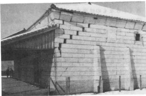
Fig. 12. Damage to a stone-built storehouse at Kyomachi.
