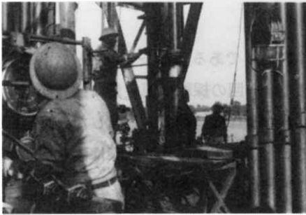
Photo. 5 A view of casing setting work
