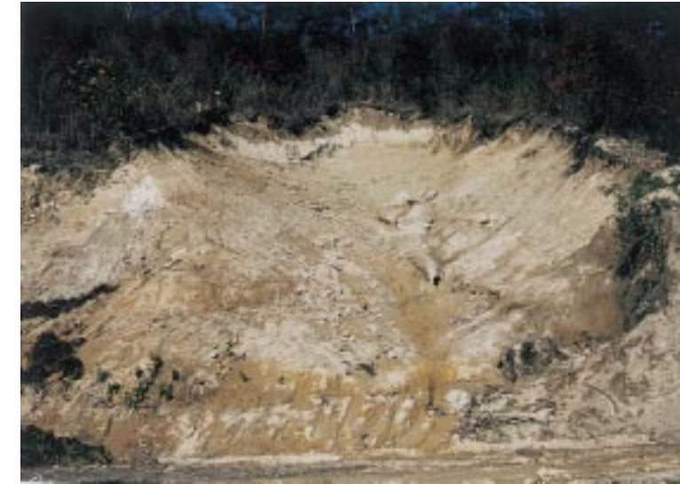
写真17 風化した白河溶結凝灰岩層中に生じた崩壊 Photo 17 Surface failure in weathered tuff.
