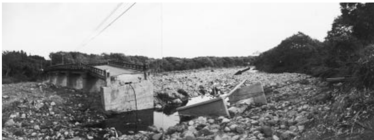
写真3 左岸側取付部が洗掘され損壊した高津橋と河床の様子 Photo 3 The left bank of the Takatsubashi Bridge was washed away.
