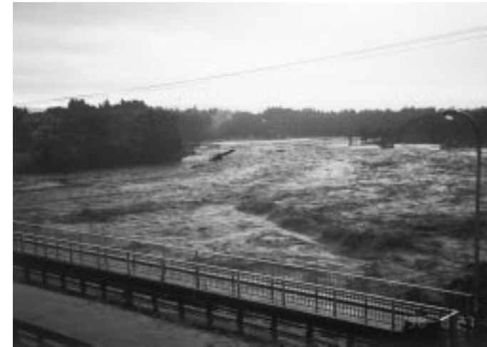
写真4.1 増水した余笹川：国道4号余笹橋 [栃木県提供] Photo 4.1 The Yosasagawa river swollen by the flood at the Yosasagawa bridge, Route 4.
