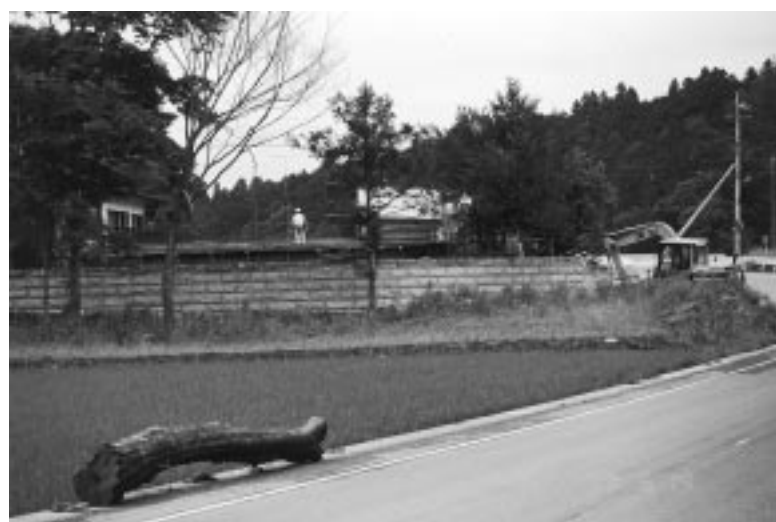
写真8.8 被災住民の水害への防備：上流側への強固な塀の建設 Photo 8.8 Solid walls behind a house as a countermeasures for flooding.
