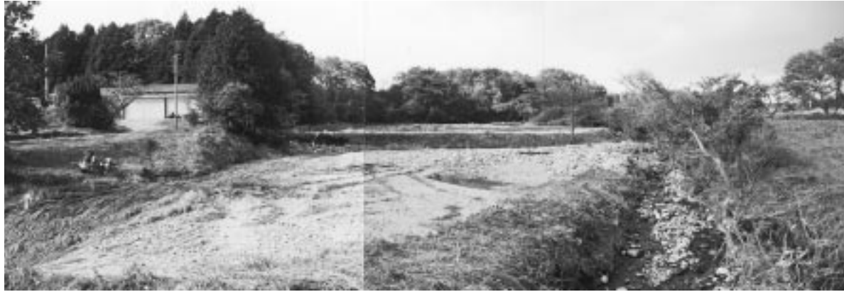
写真5 余笹川中流部：水田への土砂散乱状況 Photo 5 Sediment spread onto rice fields in the middle reaches of the Yosasagawa river.
