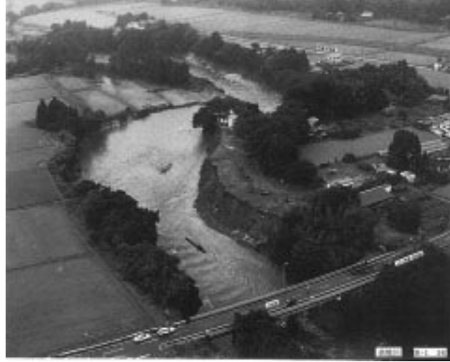
写真10.1 余笹川最下流部：造成地（左岸側）の流失 [ 栃木県提供 ] Photo 10.1 Reclaimed land on the left bank was eroded by the 1998-flood.
