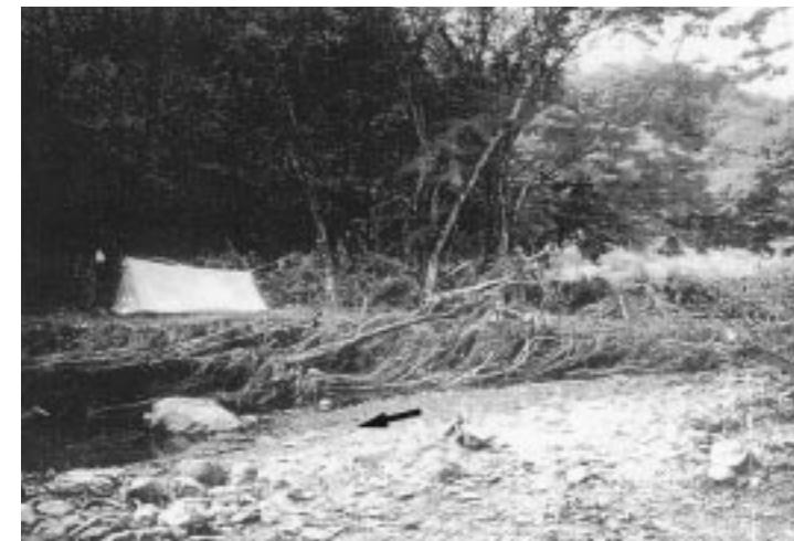
写真2.1 多羅沢川沿いの別荘地被害状況：別荘地を横切る洪水流路 (T1地点) [栃木県提供] Photo 2.1 Cottage area along the Tarasawagawa river stricken by the flood: site T1.
