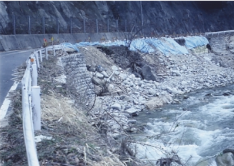
写真 13b 平谷川溪岸の侵食状況 Photo 13b Erosion disaster along the Hiratani river.
