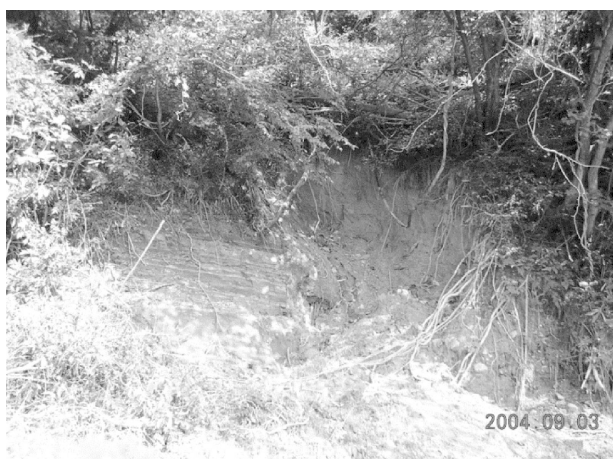
写真 2 浅い斜面崩壊（左）と深い斜面崩壊（右）が隣接していた例．栃尾市土ヶ谷近郊 Photo 2 Shallow landslide (left) and deeper landslide (right) at Tsuchigaya, Tochio City.
