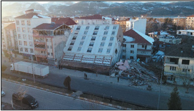
a) Damaged buildings in Golbaşı
