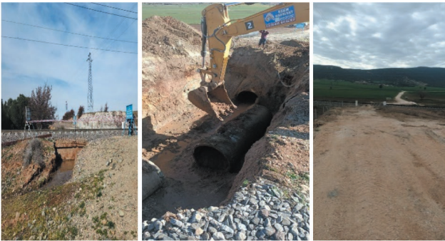
Fig. 2 Kartalkaya Pipeline Damage Repairs (Courtesy of GASKI).
