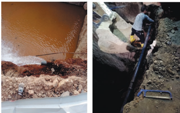
b) Operation of Repair of PVC Pipe
