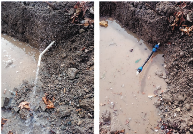
a) Blinding Operations at Destroyed Buildings
