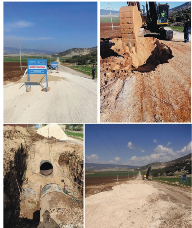
Fig. 4 Kartalkaya Pipeline Damage Repair Operations.
