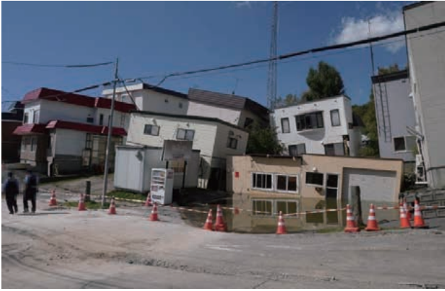
図11 札幌市清田区の液状化(撮影日9/17) Fig. 11 Liquefaction of Kiyota-ku, Sapporo (shooting date 9/17).
