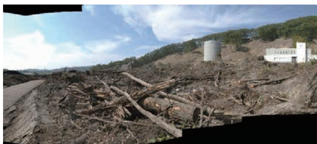
図4 厚真町の豊里浄水場周辺の崩壊現場(撮影日9/15) Fig.4 Collapse site around Toyosato water purification plant in Atsuma (shooting date 9/15).
