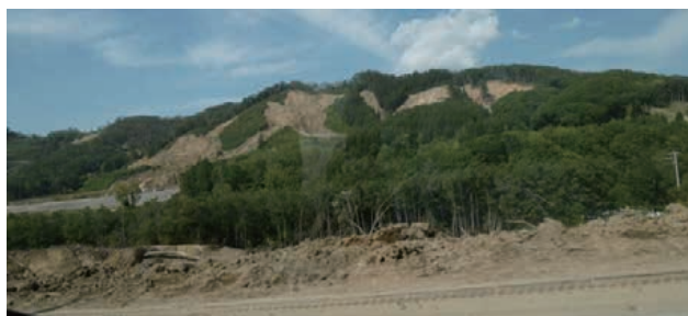
図5 厚真ダム周辺の斜面崩壊(撮影日9/15) Fig.5 Landslide around Atsuma Dam (shooting date 9/15).
